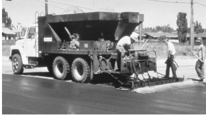
Figure 3: Slurry Seal application ( www.fs.fed.us/eng/pubs/html/99771201/99771201.htm )
